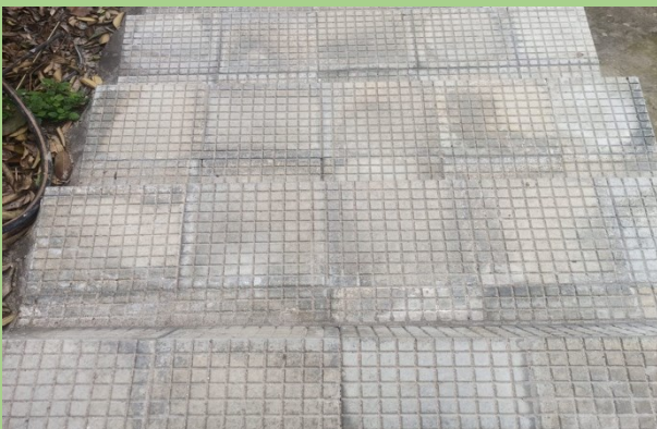
Tiling work at the Staff Quarters
