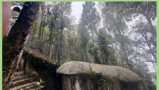
Vertical Fencing extension & Electric fencing installation at old Conservation Breeding Center
