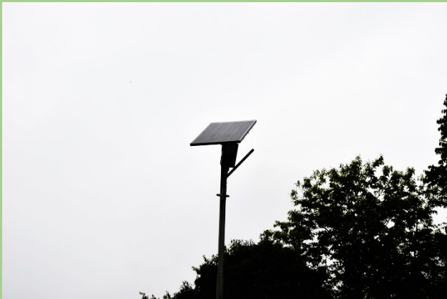
Installation of solar-powered streetlight
