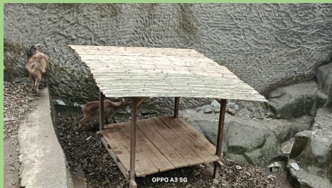
Installation of Rain shelter at Himalayan Tahr enclosure
