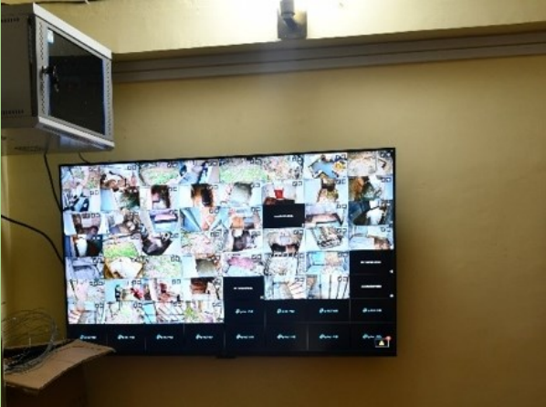
Installation of CCTV monitoring system
